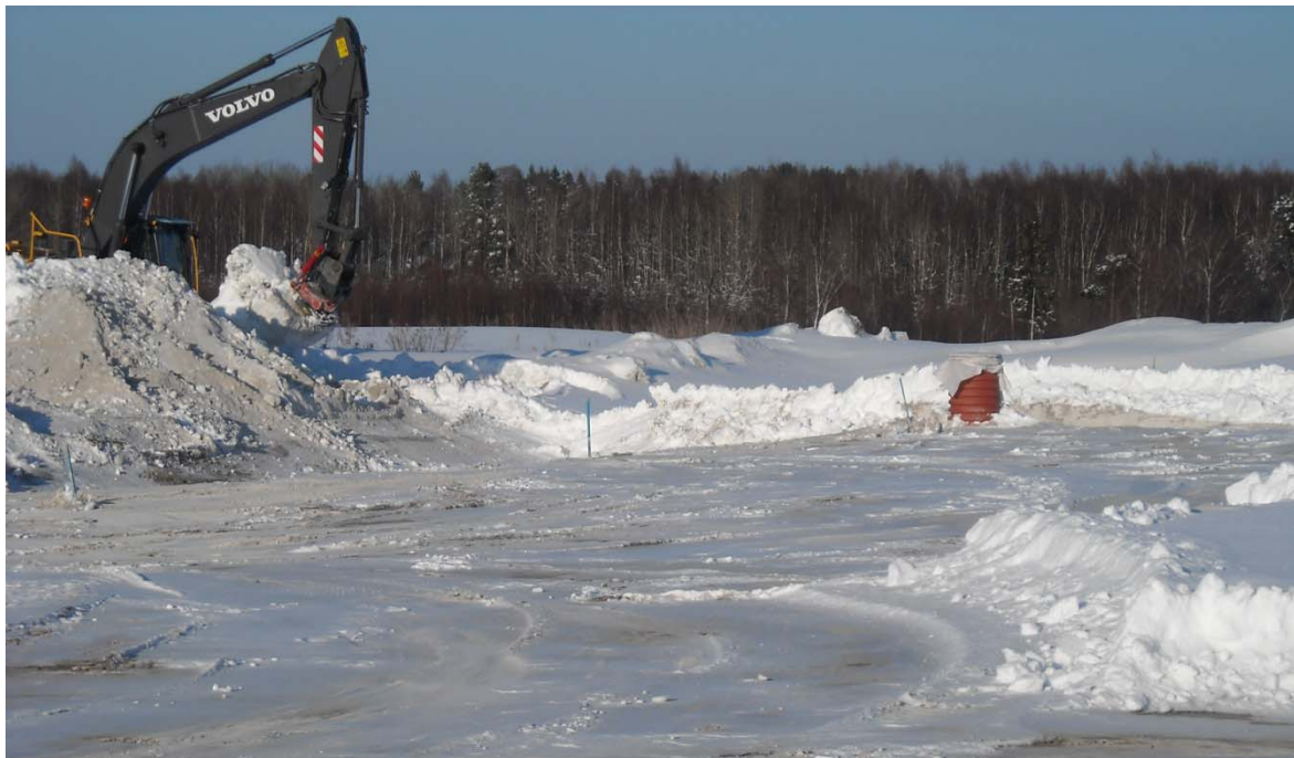
Picture 3 Snowy day during construction of the pilot surfaces.
