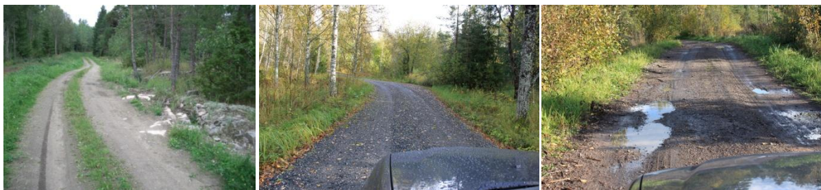
Figure 9 Ehnsjövägen, a) before stabilization (2004), b) five years after stabilization (2009) and c) a typical reference road section 2009.
