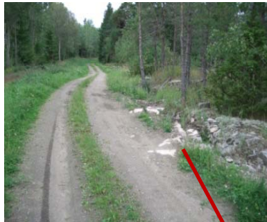
Road section 1 (2004 – before stabilization)
